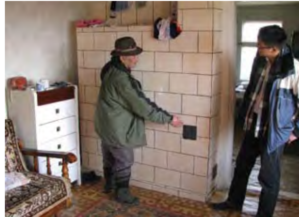
Back Side of Heating Wall
