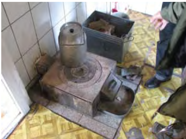
Stove with Heating Wall
